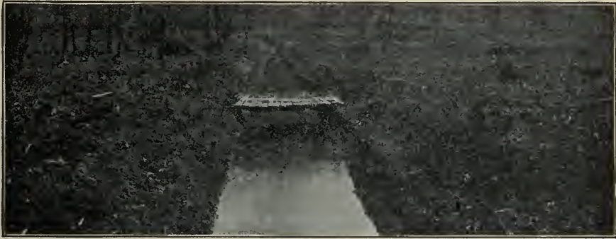
FIG. 17. — An open ditch dug through a swamp in order to drain off the water.
